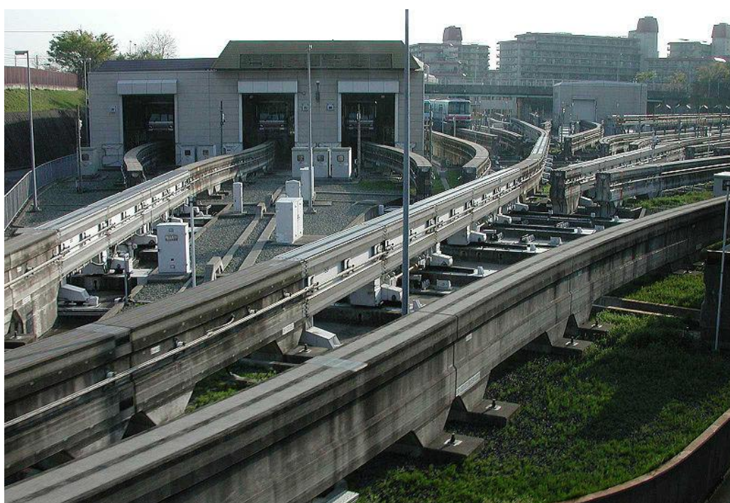
Fig. 5 Example depot in Osaka, where it is possible to move the track into several branches. They move to a bright long stretches.
