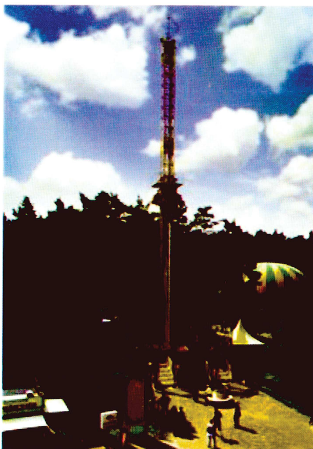
Figure 7 Drop tower, (44m), amusement ride utilizing ECB's. slika 7 Džinovski tobogan (44m), primena ECB sistema za vožnju u zabavnom parku
