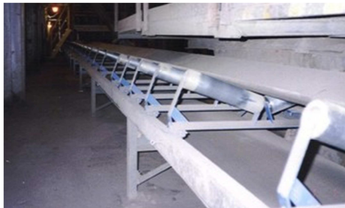
Fig. 7 Belt conveyor M21
