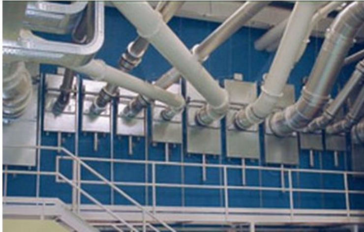
Fig. 9 View of part of pneumatic post in the hospital (source: Google Images, Stöebich Fire
